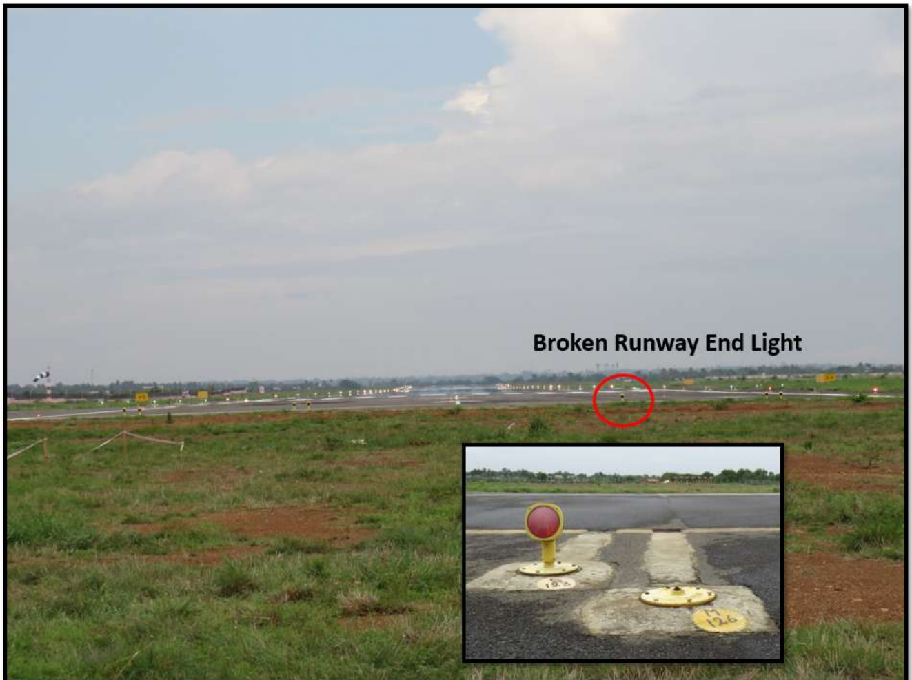
Broken Runway End Light
