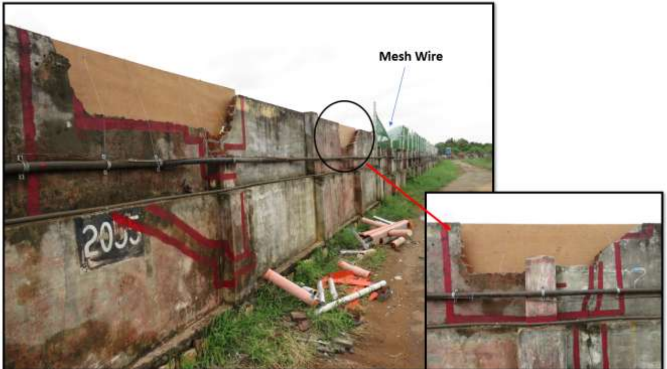
Broken Boundary Wall Portion after impact
