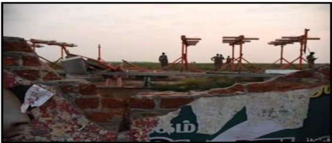
Broken Boundary Wall Portion after impact
